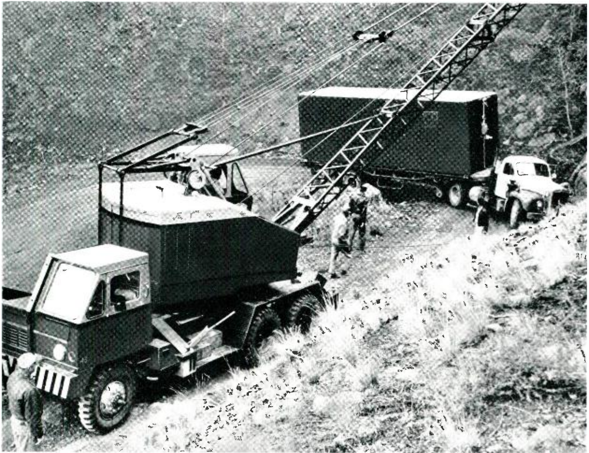
Truck transporting a packaged building for a TJ radio-repeater station must wind up mountain
