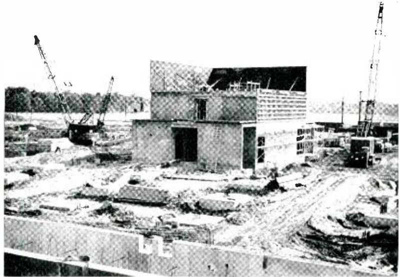
Above, an elevator shaft takes shape at the Holmdel Laboratory.
