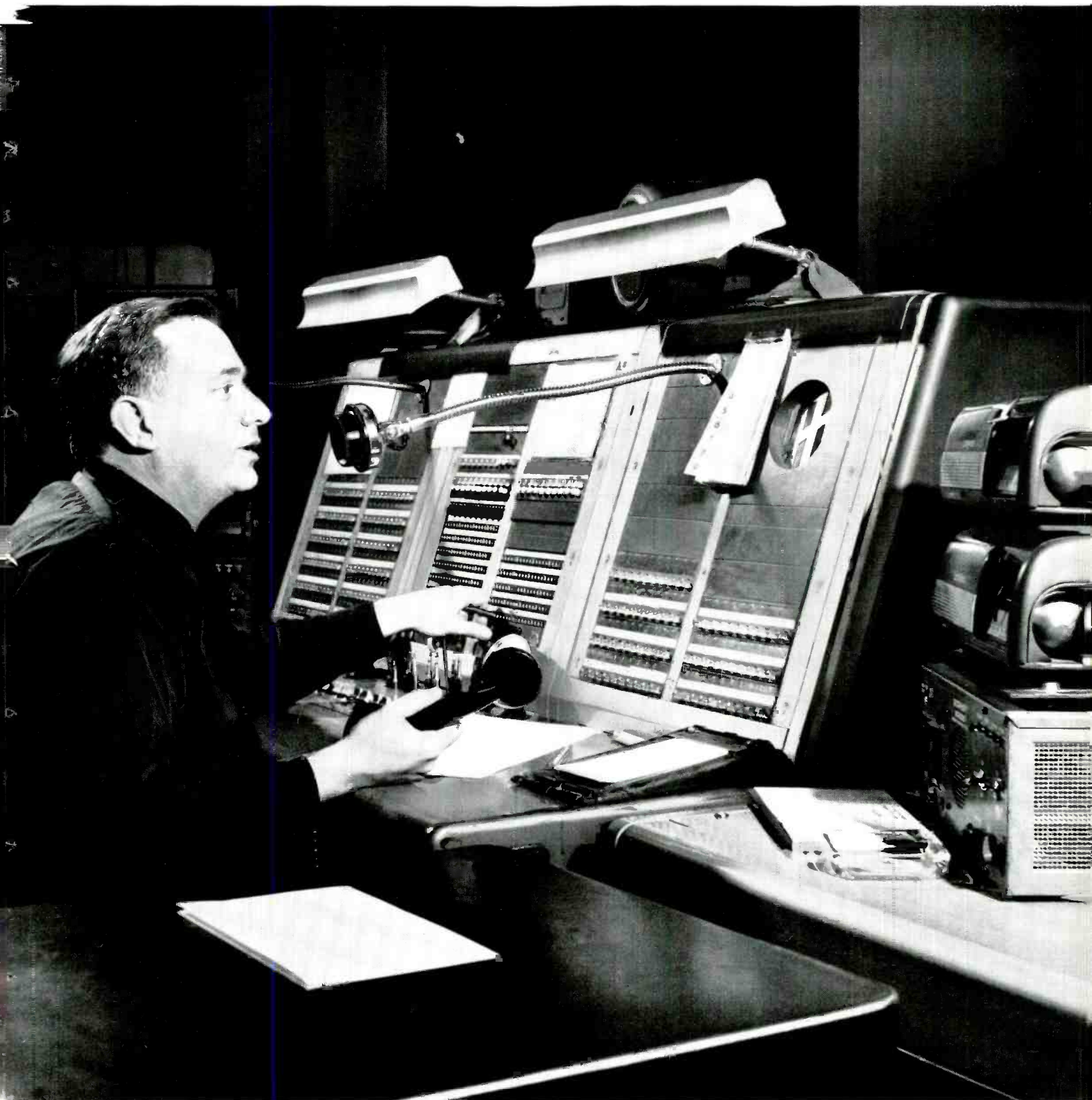
Headquarters attendant answers call at switchboard of direct-line installation at North Bergen, N. J.
