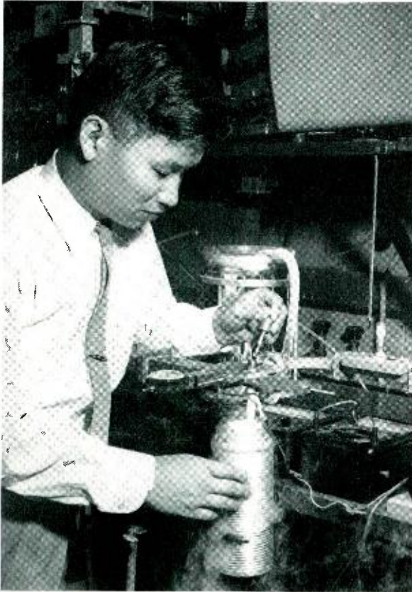
M. Uenohara inspecting diode waveguide apparatus used in work on parametric amplification.
