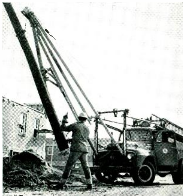
Auger and derrick are powered from truck engine. Truck-mounted derrick swings the prepared telephone pole swiftly and gently into place with no additional strain on two-man crew. These studied innovations help to speed and safeguard work.
