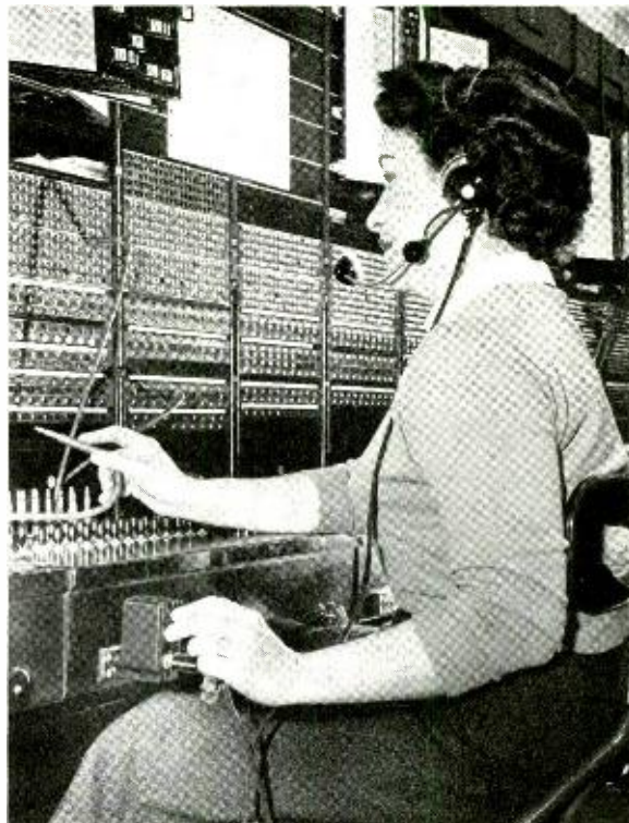
The new headset amplifier in actual use. Mrs. R. Dixon is adjusting by feel the gain-control knob. Final design of the amplifier unit was chosen only after trials to determine the best model.
