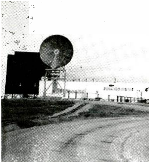
A typical White Alice station at Kotzebue, 30 miles above the Arctic Circle. At left are a 60-ft. and a 30-ft. antenna. Not shown are the two antennas for reception from the opposite direction.
