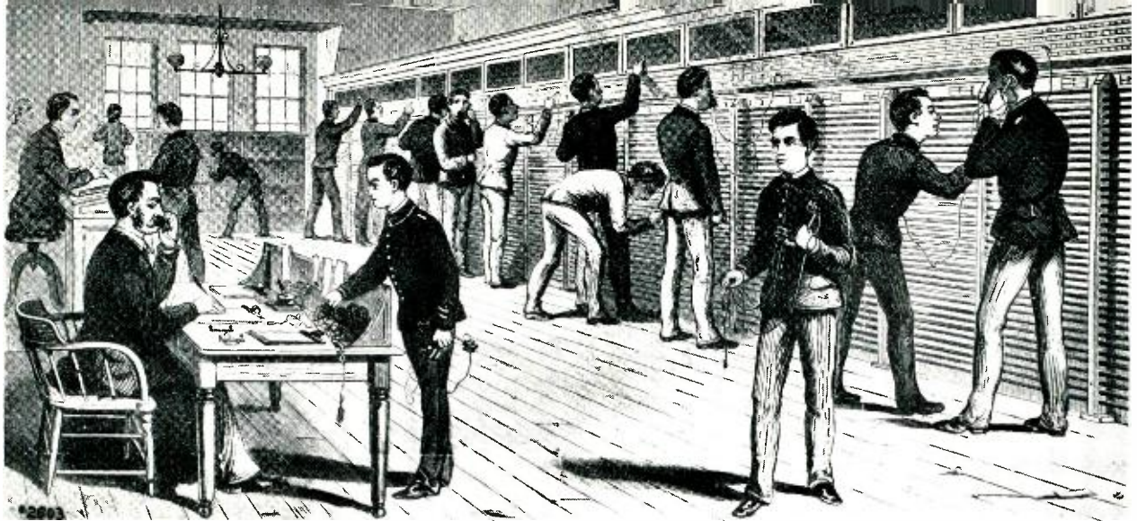
One of the earliest telephone exchanges (New York City, 1879) gives measure of eighty years of progress when compared to modern automatic systems. Need for automatic switching was recognized early.
