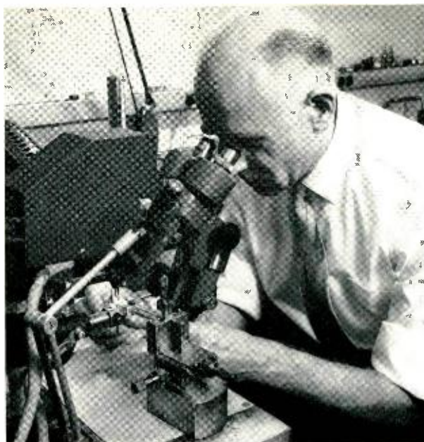
Fig. 2—E. F. Elbert performing intricate welding operation in laboratory assembly of wafer units.
