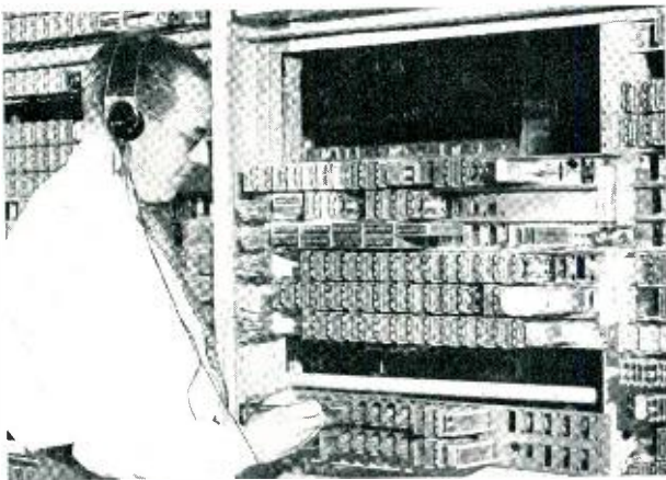
Fig. 1 — E. F. Weight, wire chief of the University office at San Diego, does some final checking on new senders just before the cutover.
