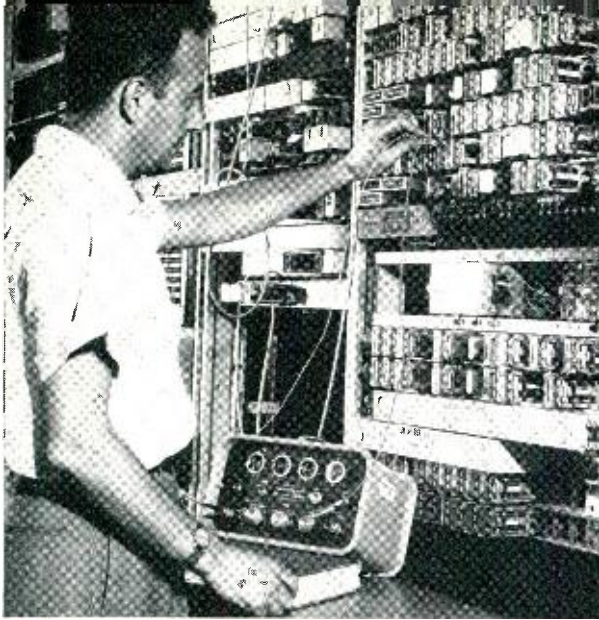
Fig. 3—A. P. Famiglietti measures the operate time of a relay in a C.A.M.A. incoming register.
