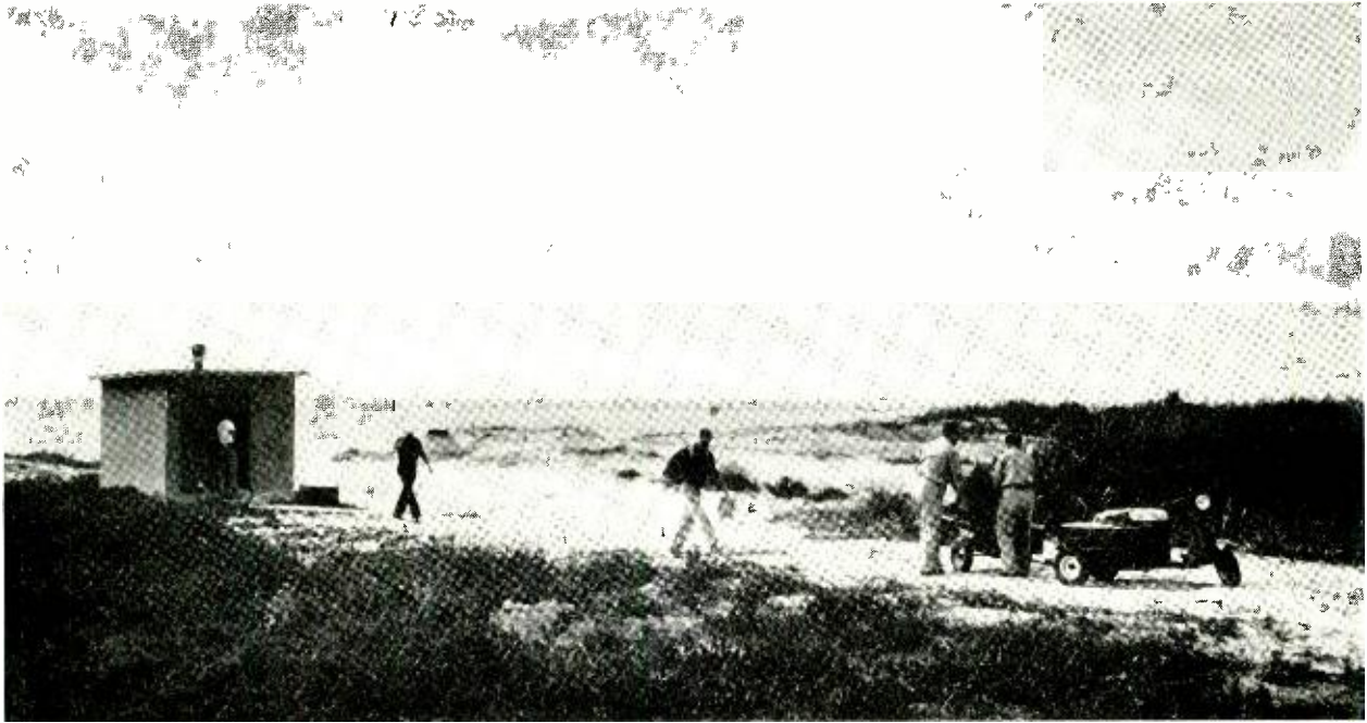
Fig. 2 — A filter hut, part of an unattended repeater, on one of the island sites.
