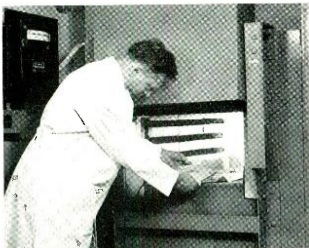
Fig. 6—H. D. Cook prepares to fire the silver electrodes on an ultrasonic delay line.
