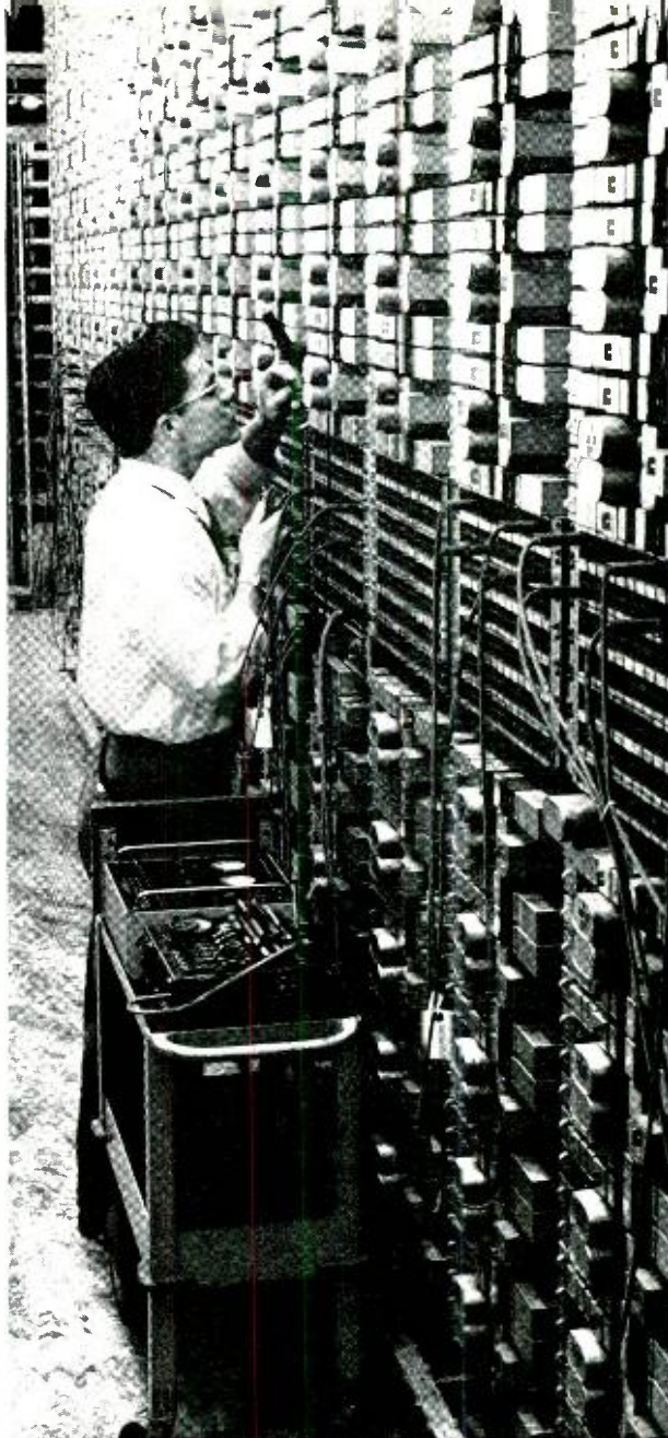
Fig. 3 — D. J. Collins, Long Lines equipment maintenance man, adjusting the sensitivity of 1A echo suppressors in a New York toll office in the Long Lines Building.
