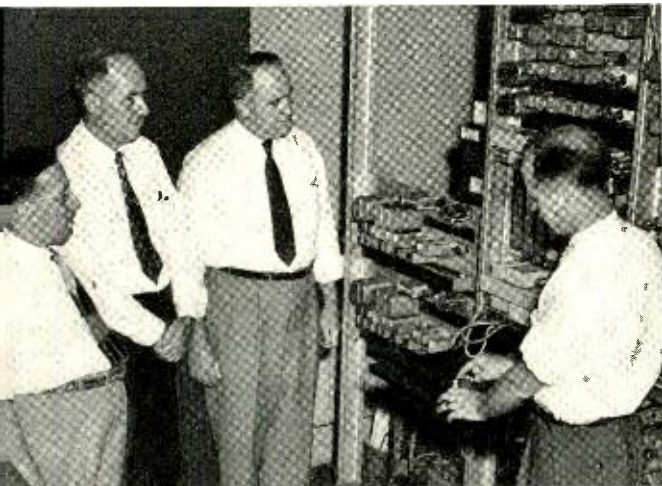
Considerable interest has been shown by Telephone Company people in the warning system. One group which visited the Laboratories recently to see and discuss the system consisted of James Poole, A. A. James and E. P. Hurley, all of The Southern New England Company.
