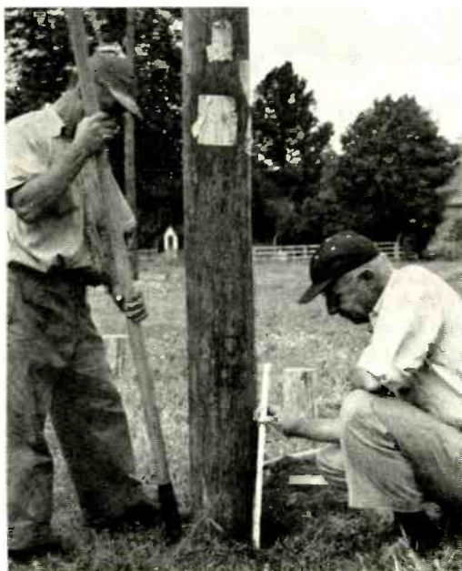
Bill and Wayne Parks check pole stubs having special preservative treatment.
