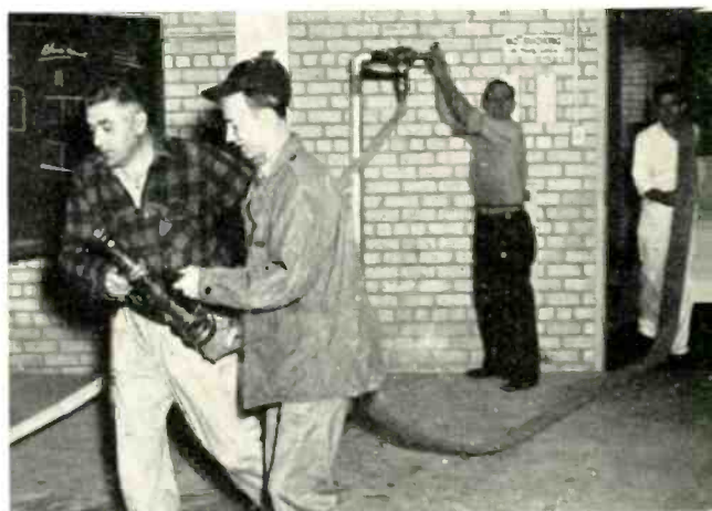
Holding a fire in check with a house line, the men in the foreground are stretching in a "city" hose connected to a stand pipe on the floor below.
