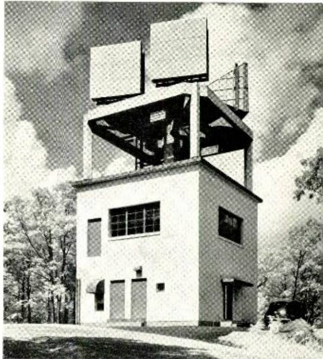
Fig. 3—Modern microwave radio station on the New York-Boston relay system.
