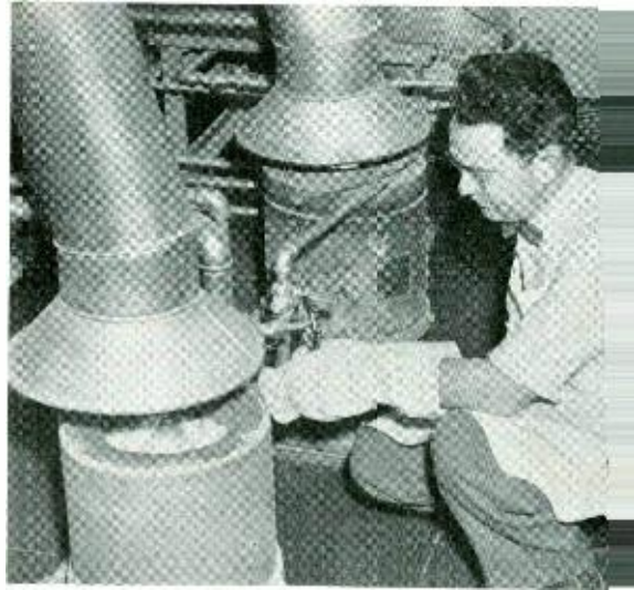
Fig. 4—Gas-fired pot furnaces used for test firings
