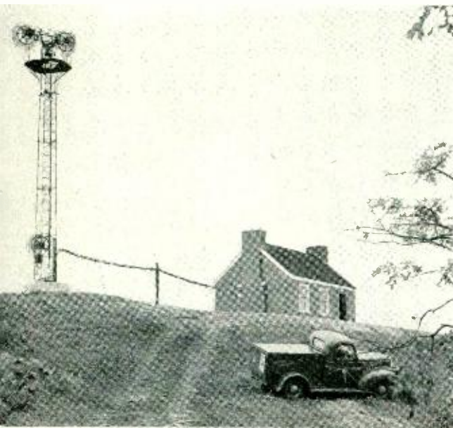
This microwave radio station at Barnstable on Cape Cod provides eight channels between there and Nantucket
