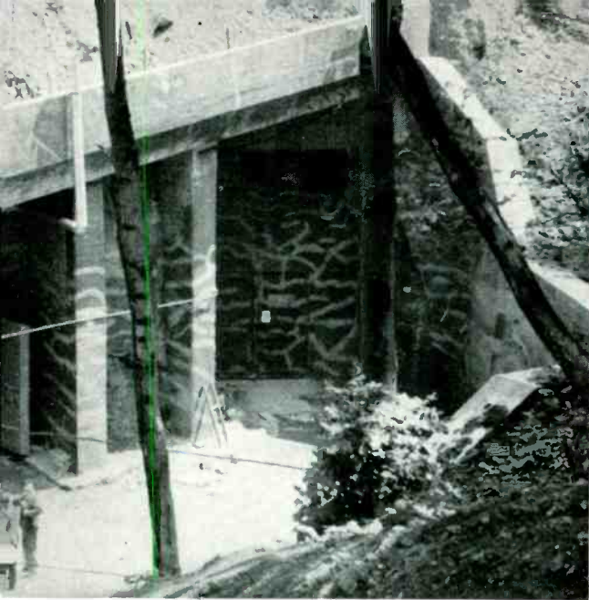
Entrance to an underground plant; the embankment that is shown in the foreground is to prevent skip-bombing
