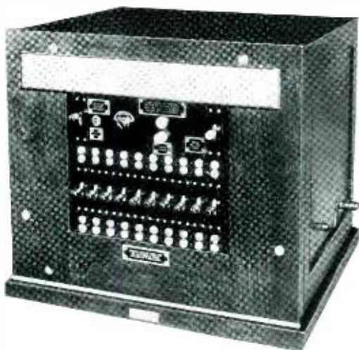
Emergency reporting switchboard of the turret type with twenty-line capacity
