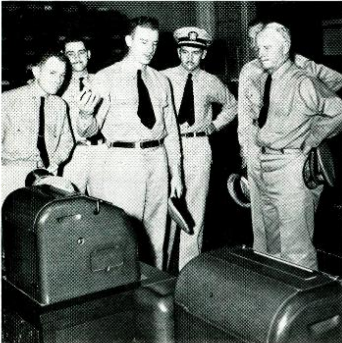
Admiral Nimitz inspects apparatus of B. T. L. design for the recording of electrical data taken at the rate of 40 observations a minute. Each observation involves a balancing operation. Results are recorded on a teletypewriter
