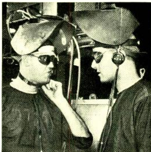
Throat microphones used in the training of student welders
