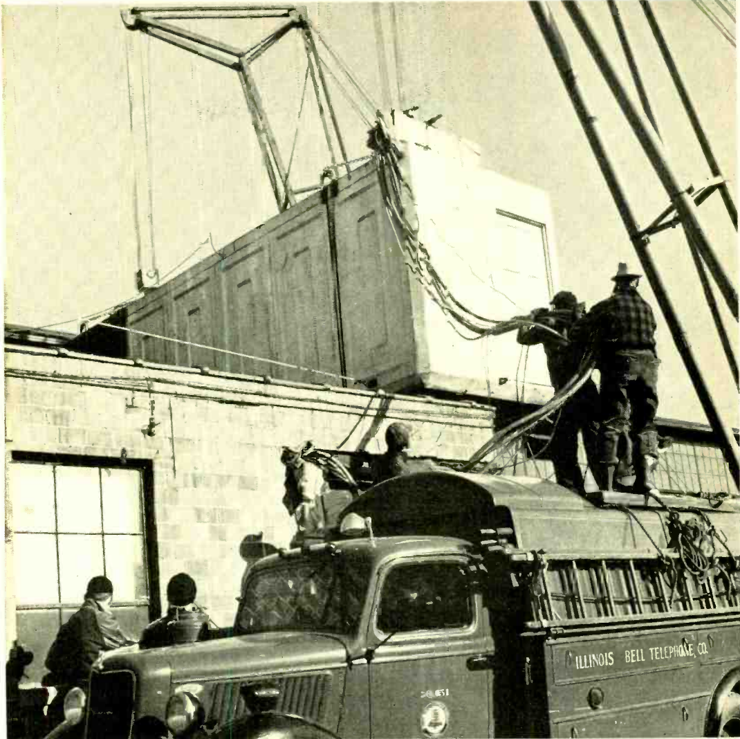
As Illinois Bell men guard the cables, a metal building housing a dial PBX is lifted to a rooftop without interrupting service
