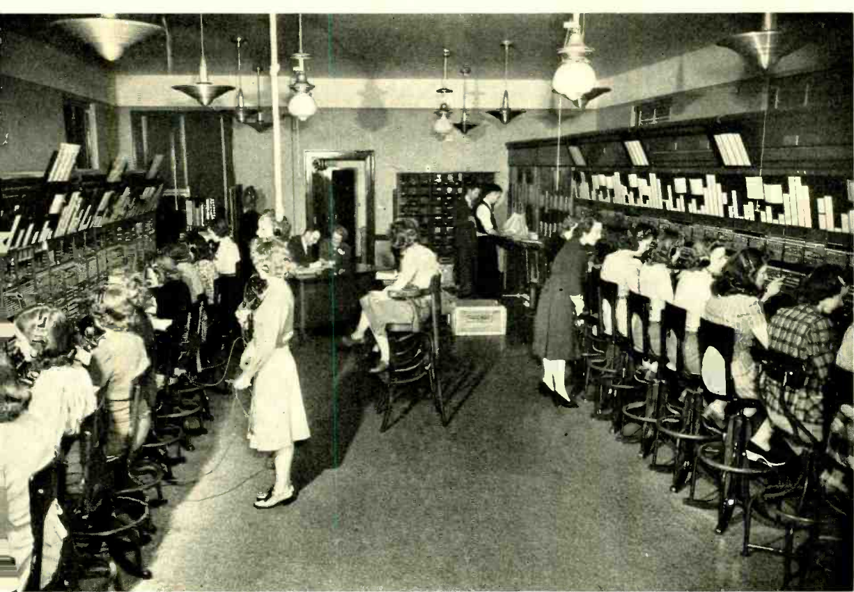
The expansion required for telephone service to an Army camp is well illustrated by the history of the Mt. Holly, New Jersey, Central Office. Twelve positions have been added to the original ten and twelve more will shortly be in service
