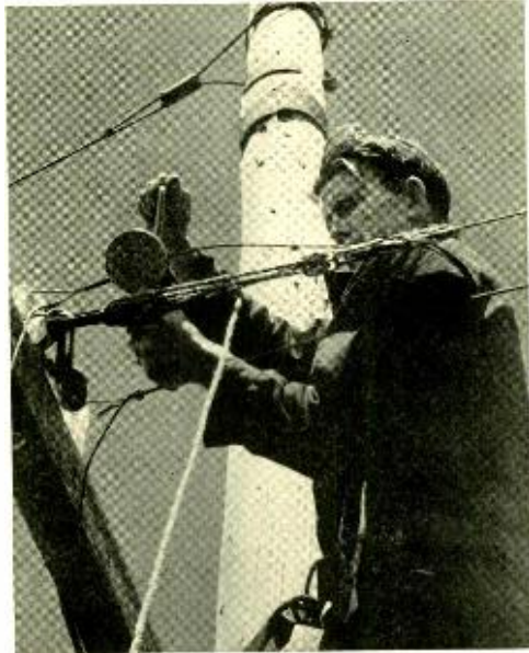
Fig. 3—Rolling the sleeve to the wires with a rolling tool
