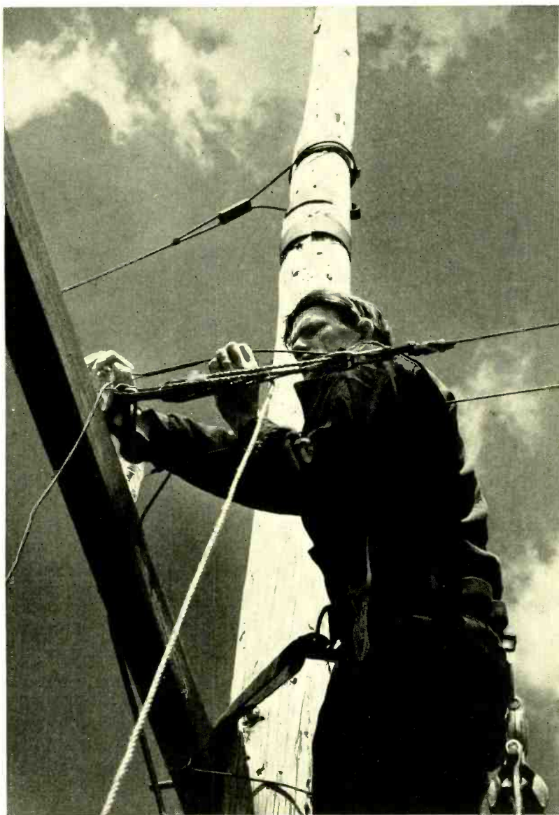
Dead-ending open wires with a rolled-sleeve joint.
