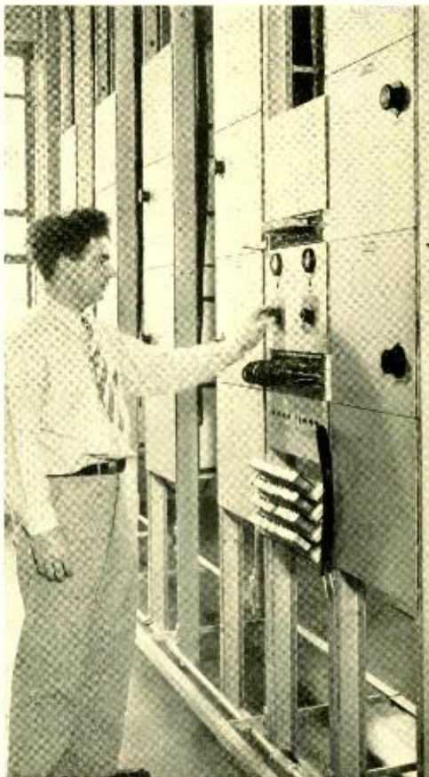
Fig. 1—The line patching panel is in the middle of the first row of bays, which comprises the input filters and first detectors
