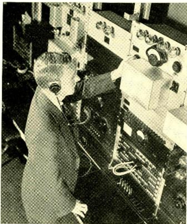
Testing toll circuits with a return-loss set which measures the unbalance between a line impedance and a network impedance. When the return-loss is high the balance is good and this condition makes two-wire repeatered circuits operate most satisfactorily
