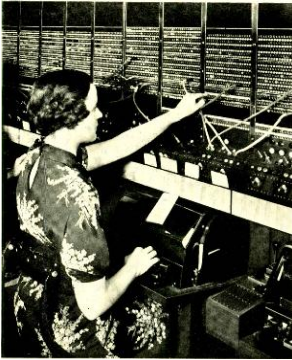
Fig. 3—In the 1A board there are no answering lamps for the trunks, and the teletypewriter is below the keyshelf on a table with a sloping top
