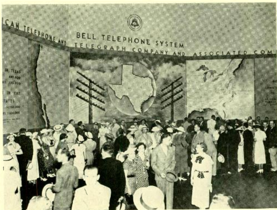
One end of the Bell System exhibit at the Texas Centennial Exposition. Along the side of the wall are placed telephone receivers through which guests are listening to a demonstration long-distance telephone conversation. The architectural plans and the apparatus which are exhibited were developed in Bell Telephone Laboratories. The exhibit is operated by the Southwestern Bell Telephone Company
