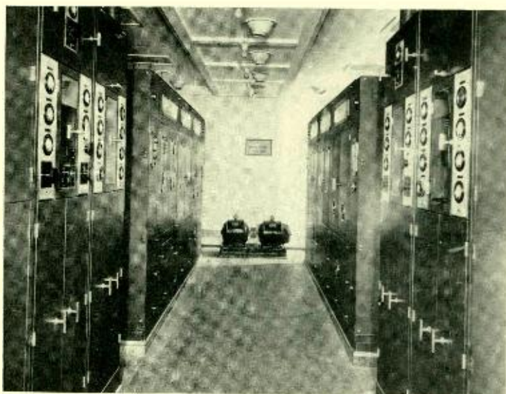
Radio room of the Queen Mary showing her two high-frequency transmitters, supplied through the International Telephone and Telegraph Company
