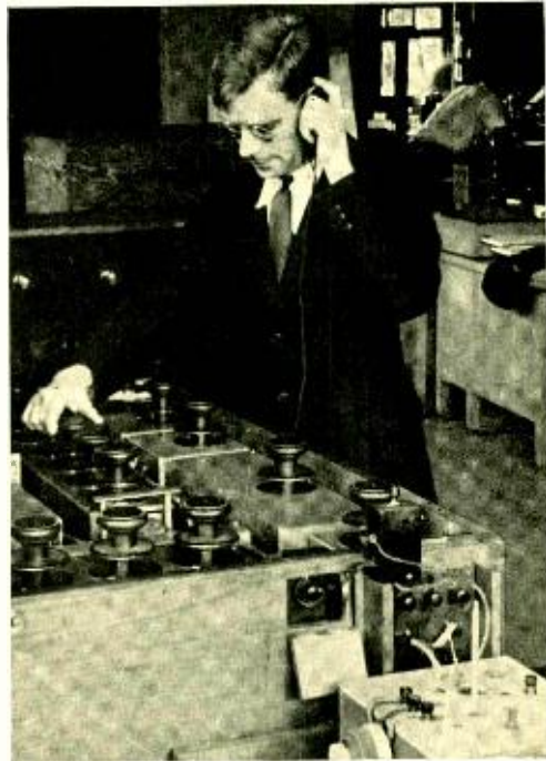
Fig. 3—Measuring dielectric characteristics
