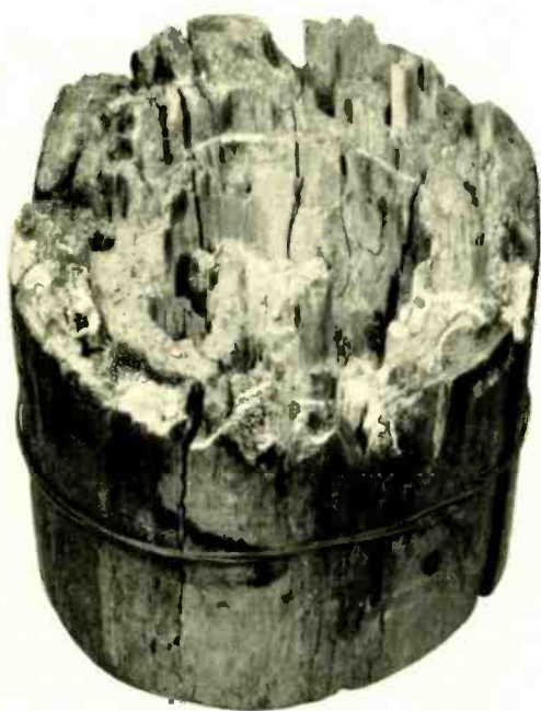
Fig. 5—Chestnut poles occasionally rot across the whole diameter. Rots of this type cannot be controlled by treating the butts of the poles with creosote because the infection works from the inside out
