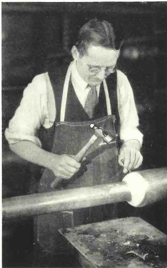
Fig. 5—Stamping the splicer's number on a finished joint
