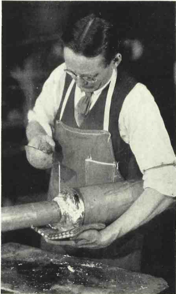
Fig. 3—Molten lead is poured over the joint to heat it to the proper temperature and to supply the metal for the wiping process
