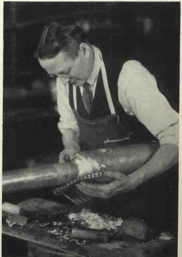
Fig. 4—The metal in plastic form is wiped to the proper shape with the "catch cloth"
