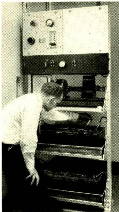
Fig. 5—A power plant forms one of the three units of the No. 12 board
