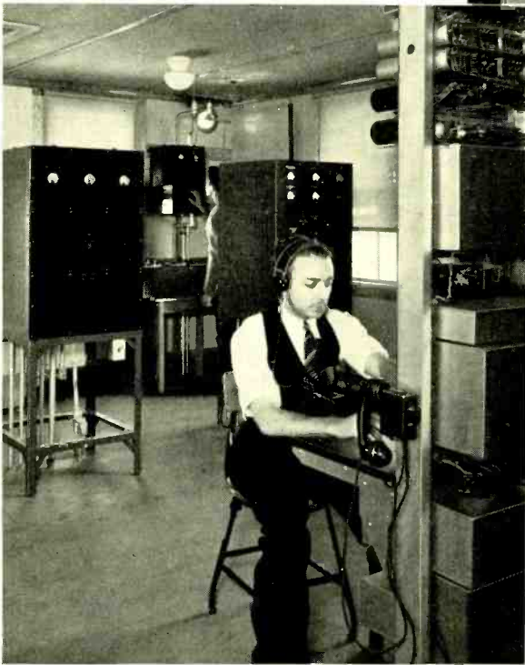
Fig. 1—Shore station at Green Harbor with J. M. Henry, who supervised the installation, at the voice-frequency control equipment
