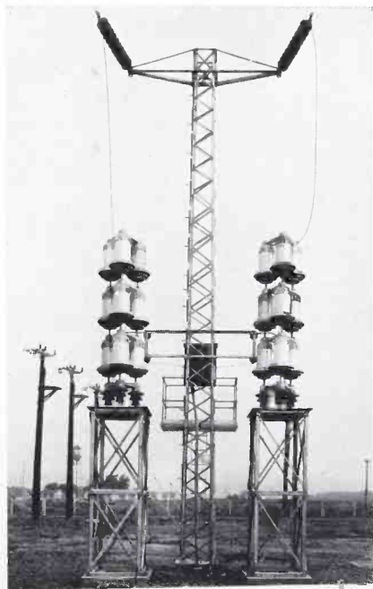
Fig. 6 — 110,000 volt coupling equipment at Newark Substation
