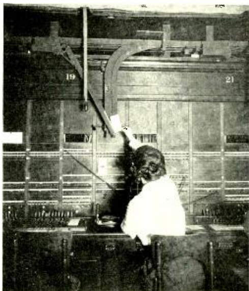
A line operator places the completed ticket in the hoist
