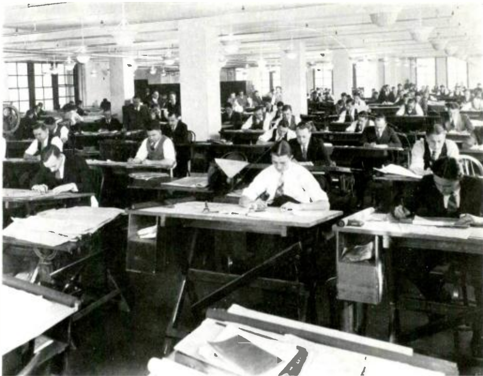
The new Systems Department drafting room on the fifth floor of Section 11
