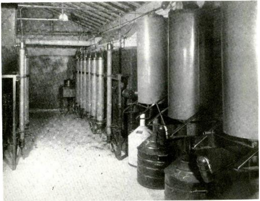
Fig. 2. From the compressor the air is piped to this room to be purified and liquefied. The liquefiers are in the foreground
