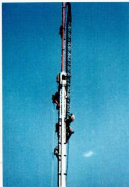
Workers installed a Dielectric NTSC directional antenna for WHSE-TV on the Empire State Building in 1990.
