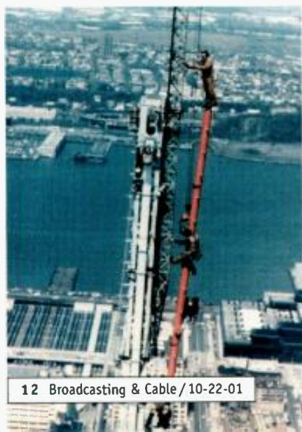
Workers installed a Dielectric NTSC directional antenna for WHSE-TV on the Empire State Building in 1990.
