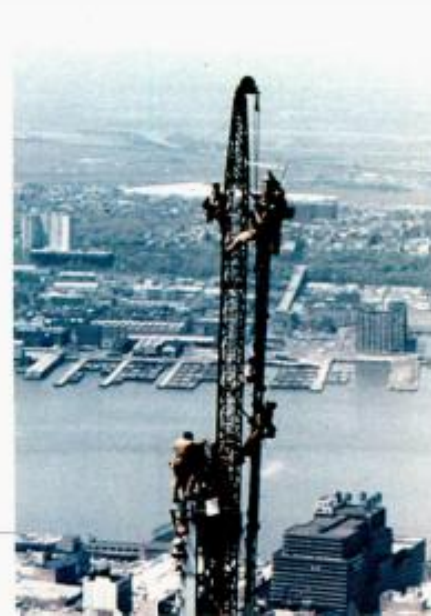
Workers installed a Dielectric NTSC directional antenna for WHSE-TV on the Empire State Building in 1990.
