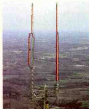
Andrew's Stacker allows one station's antenna to be serviced or swapped out with interfering with another station's performance.
