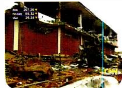
CNN delivers pictures of damage from Thursday's missile strike in Khartoum.
