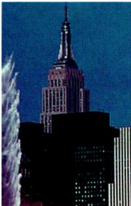
WCBS-TV's wideband antenna atop the Empire State Building may serve as an interim solution for broadcasters looking for a DTV transmission site.
