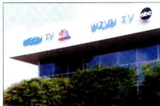
Waterman Broadcasting's Fort Myers, Fla., facility houses both WBBH-TV (NBC) and WZVN-TV (ABC).
