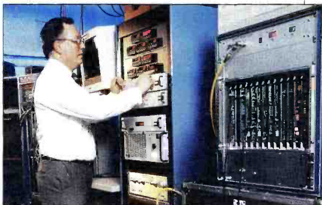
A Grand Alliance engineer makes final adjustments to an HDTV transmitter.
