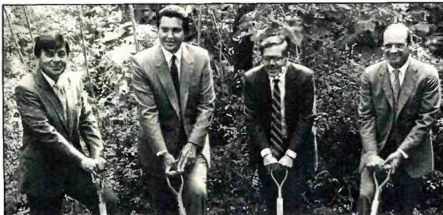
Under construction. Taft Broadcasting's wcix-TV has begun construction of its $6-million communications center, to house offices and broadcast facilities of the Miami independent. The center is expected to be completed in July 1985. Shown above at groundbreaking ceremonies are (l-r): Harvey Cohen, vice president and general manager of wcix-TV, Raul Martinez, mayor of Hialeah, Fla.; Ro Grignon, Taft Broadcasting executive vice president, television, and Dudley Taft, president of Taft Broadcasting.
