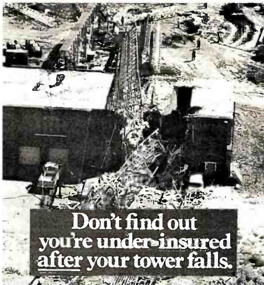
This 1375 foot, 3-station transmitting tower in Minnesota collapsed and fell across the building housing the transmitter, killing seven people.
