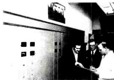
Gale Allred, Chief Engineer, with KFQD's powerful 50 kW AM transmitter notes: "It has by far the best overall frequency response I have ever seen, including distortion." Translated, this means better quality sound that encourages listeners to keep their radio dials set at 750.
