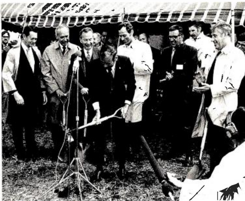
Ground is being broken by Iowa Governor Robert D. Wray for a new 2,000-foot jointly owned tower designed for common use by three Des Moines-area stations. WOI-TV, WHO-TV and noncommercial KDIN-TV will move their transmitters to the site 15 miles north of that city. Behind the governor (l-r): Wayne J. Blick, Palmer Broadcasting, parent of WHO-TV licensee; Robert H. Harter, VP and general manager, WHO Broadcasting; Dr. Robert F. Ray, chairman, Iowa Educational Radio and TV Facility Board; John Montgomery, executive director, Iowa Educational Broadcasting Network; Robert Mulhall, general manager, WOI-TV, and Dr. W. Robert Parks, president, Iowa State University.
