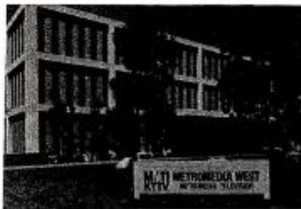
Three-story main building, of 140,000 square feet, houses studios and offices of KTTV(TV), Metrotape West and western branch of Metromedia corporation. Steel and concrete frame carries pre-cast panels of stone cast in resin.
