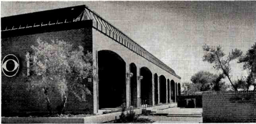
An abandoned egg warehouse provided basis for new KXTV(TV) Sacramento, Calif., studios. Renovation of dilapidated property into a "Spanish design indigenous to the Sacramento community" cost $1.3 million.
