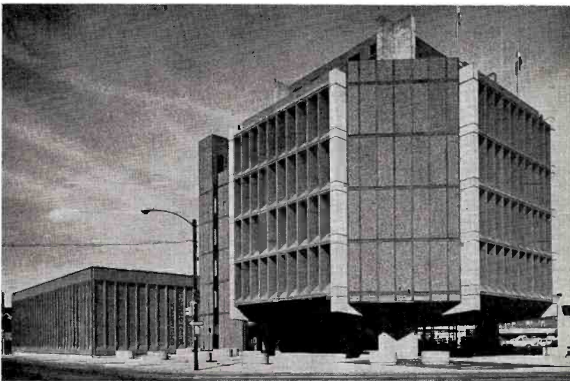
The new home of KLZ-AM-FM-TV Denver is a cantilevered five-story octagonal-shaped tower connected to two-story conventionally shaped rectangular box which serves primarily as main TV studio area. Building best reflects architect Raymond Bowers's contention that broadcasters are showing new concern for "visual identification in the community as well as on the air."
