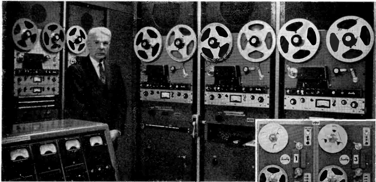
▲ Granville Klink, chief engineer WTOP-WTOP-FM., Washington, D.C., at console, surrounded by four Scully 280's and 2 280-2's in master control tape room.
