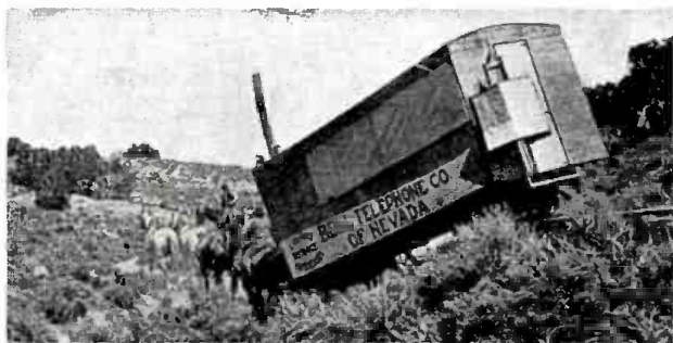
Installers of the first transcontinental telephone line had to surmount hardships of windstorm, ice and scorching heat combined with rugged country.
