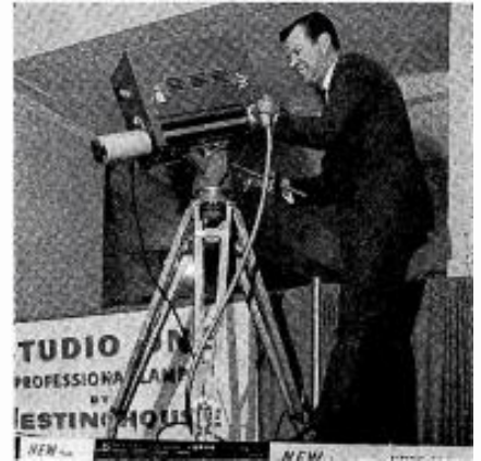
Thomson Electric's new transistorized 4-inch image orthicon camera with zoom lens.
