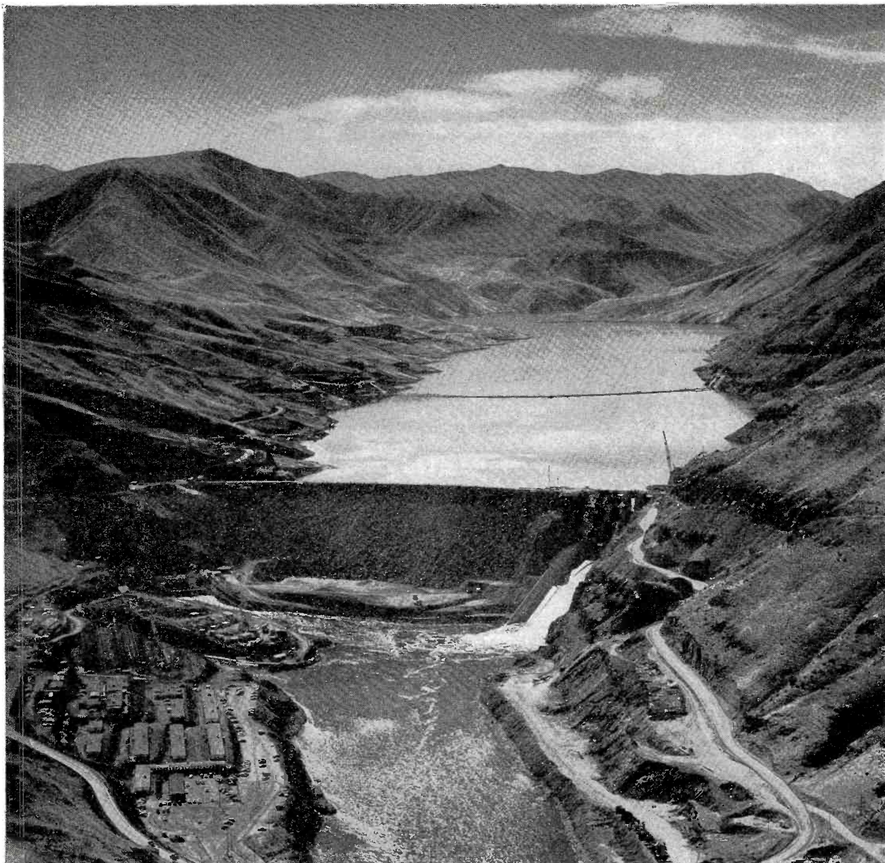
The year-old Brownlee power dam on the Snake River between Idaho and Oregon, built by the local independent electric company, the Idaho Power Company. The project embraces the Oxbow dam and the Hells Canyon dam down river from Brownlee.
