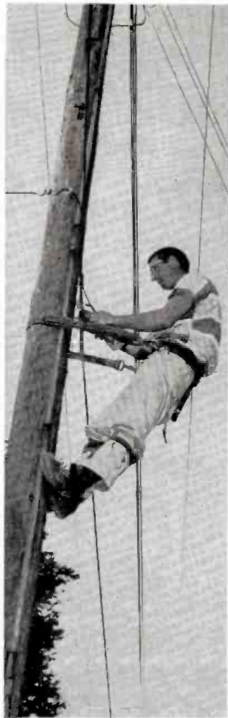
SERVICEMAN taps the home feed-in onto the coaxial trunk.
